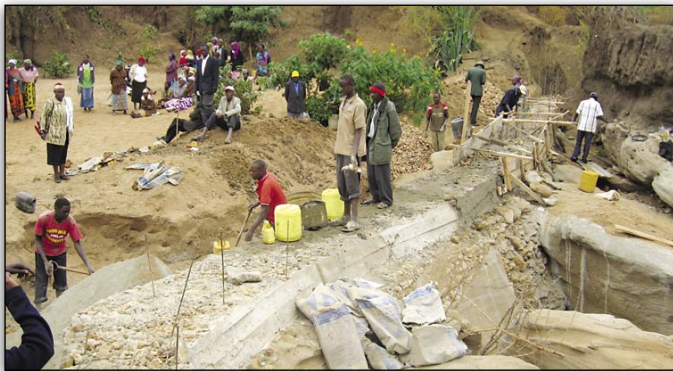
Community members building a dam
